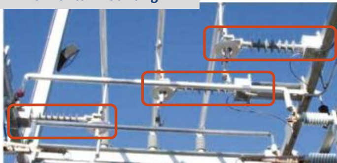
John Deer Wind Farm, USA 69 kV horizontal mounting
